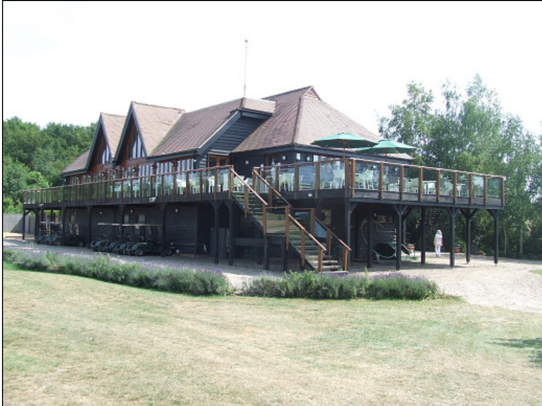
Photograph showing existing clubhouse serving Wildwood Golf and Country Club (view looking south).
