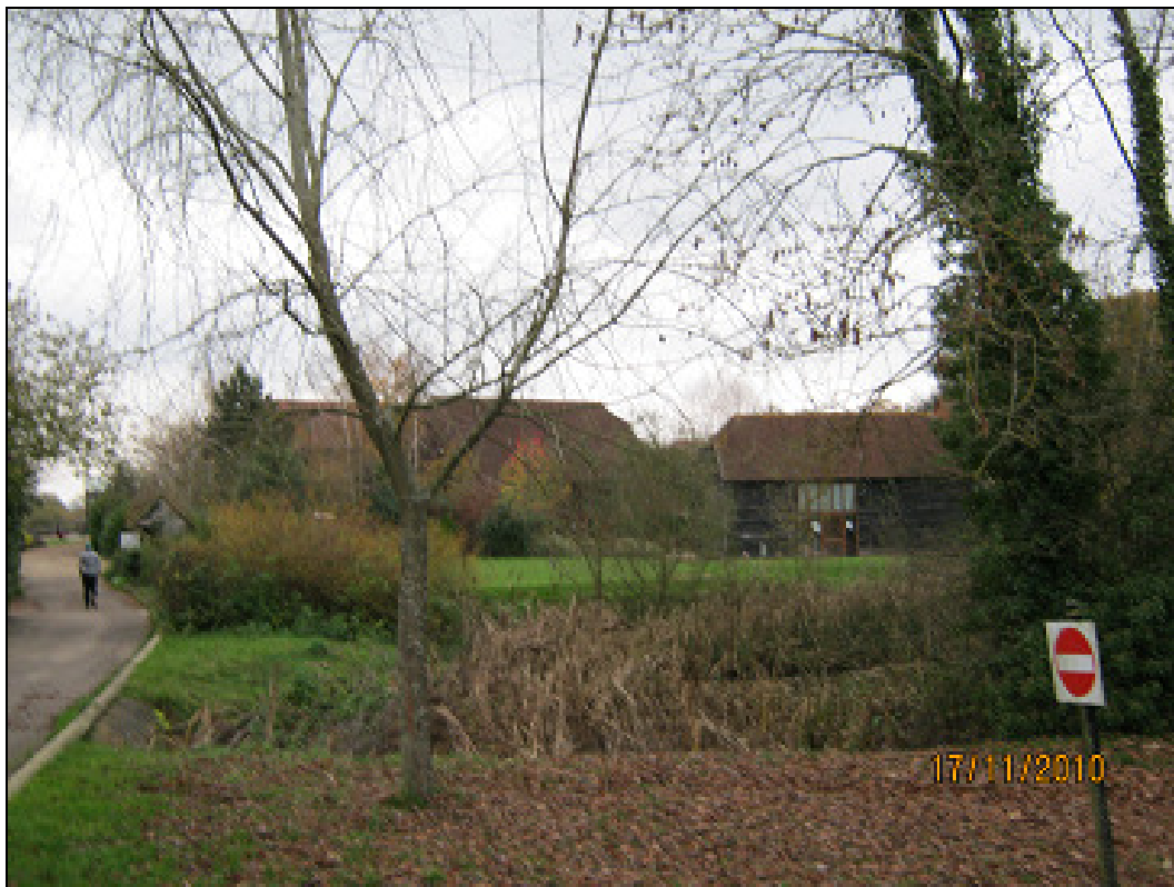
Photograph showing existing clubhouse and grade 2 listed haybarn serving Wildwood Golf and Country Club (view looking north east).
